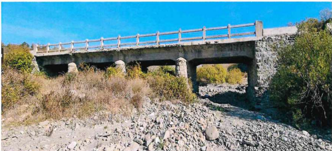
Figure 3: Selenica Bridge Nr.2 – Picture taken from the existing situation
