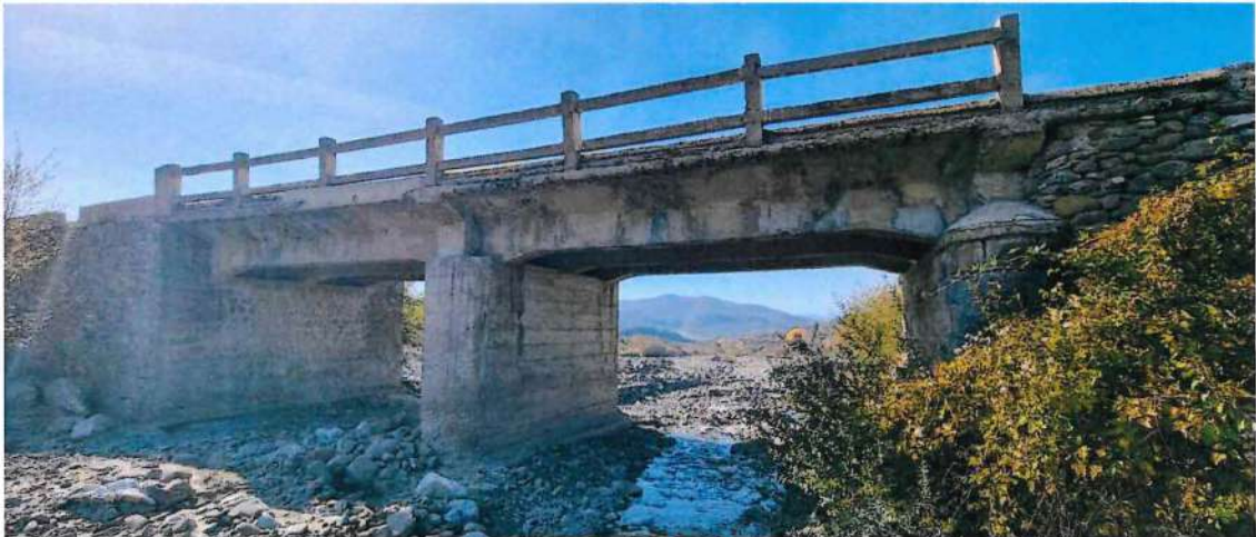
Figure 2: Selenica Bridge Nr.1 – Picture taken from the existing situation
