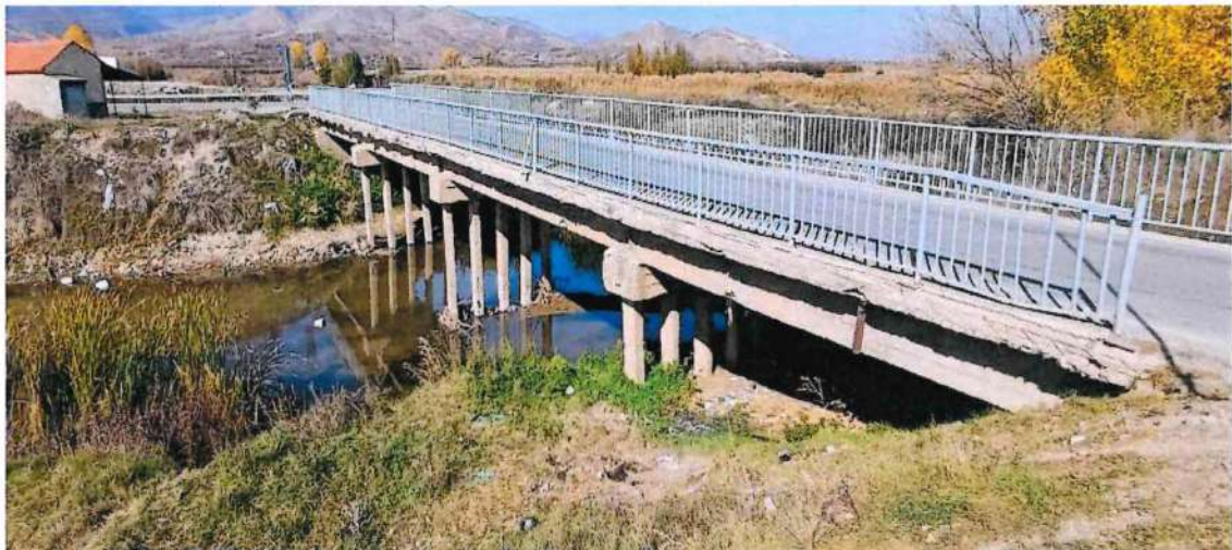
Figure 6: Turan Bridge– Picture taken from the existing situation
