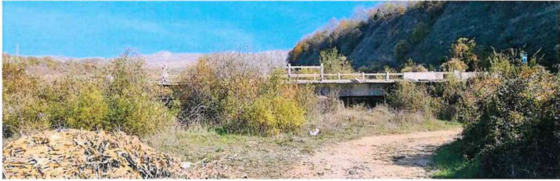
Figure 4: Selenica Bridge Nr.3 – Picture taken from the existing situation
